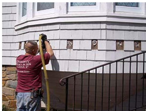
Existing above ground sidewalls are most commonly insulated by removing siding or drilling holes into the sidewall and blowing loose-fill into cavities.
